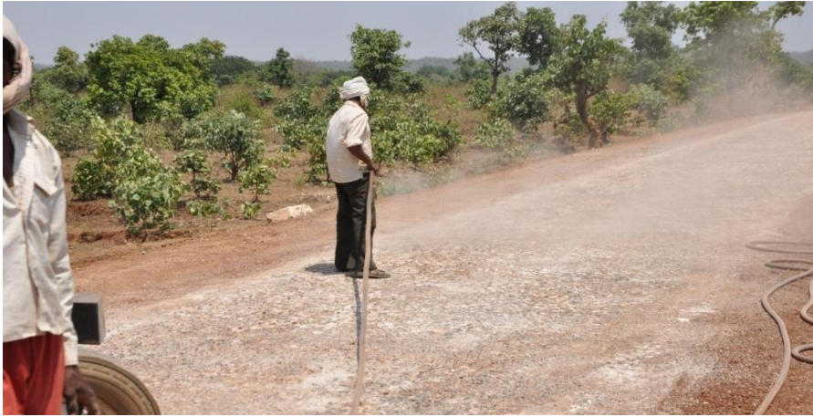
Cleaning of Gravel Surface
