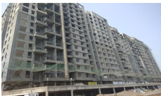
Fig 5: Plastering at site
