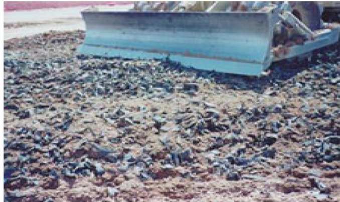
Figure: Shredded scrap tires used as road base
